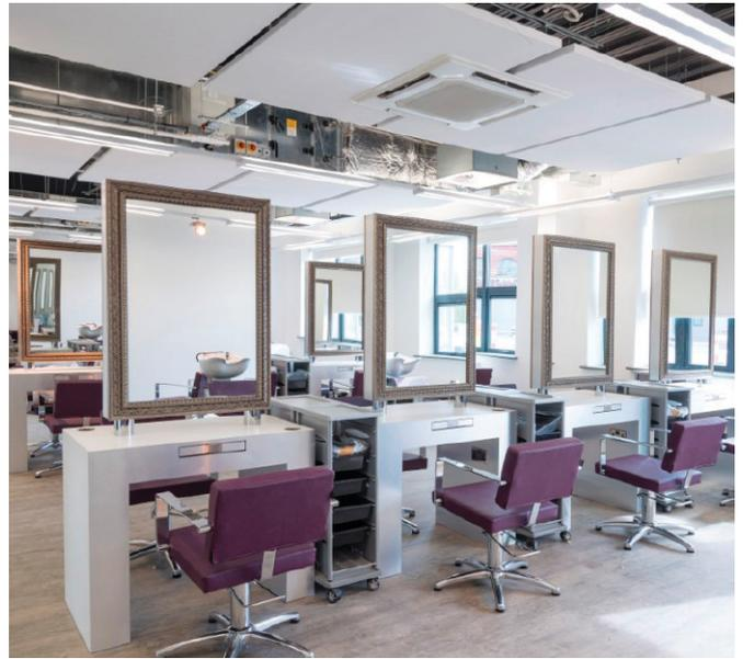
The islands are made of a 40mm stone wool panel, which is a natural sound absorber, enabling optimum acoustic comfort. The islands are elegant floating panels hung from discreet suspension wires, making them a versatile product for refurbishment projects. The visible side of the panel has a smooth white surface. The panels allow air to circulate whilst absorbing sound from both sides of the panel, which is perfect for thermal mass buildings.
